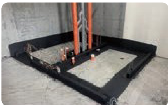
止水墩座施作
